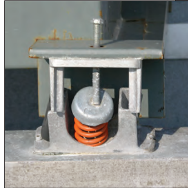
Figure 8. The equipment on this stand was resting on vibration isolators that provided lateral resistance but no uplift resistance (above). A damaged vibration isolator is shown in the inset (left).
